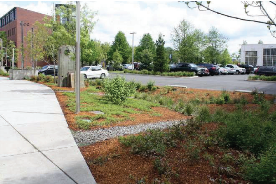
A stormwater swale adjacent to the parking lot drive aisle doubles as snow storage area in the winter
