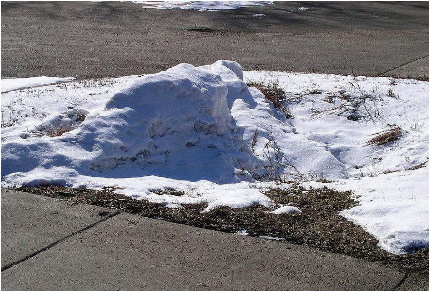
A stormwater swale adjacent to the parking lot drive aisle doubles as snow storage area in the winter
