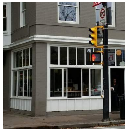
Large shop-front windows broken up using substantial trim and molding treatments
